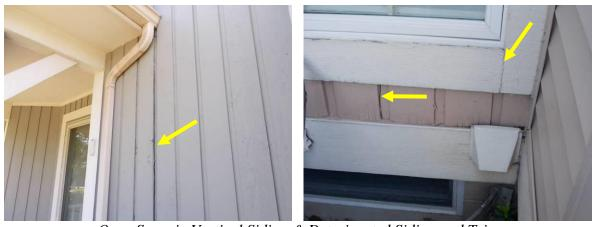
Open Seam in Vertical Siding & Deteriorated Siding and Trim
