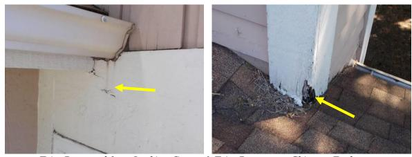
Trim Damaged from Leaking Gutter & Trim Damage at Chimney Enclosure
