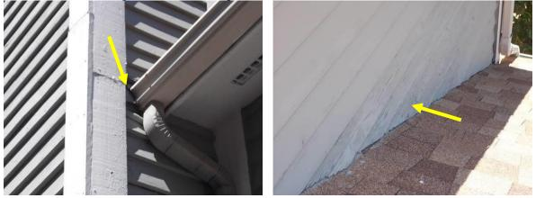
Examples of Deterioration to Clapboards
