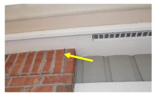
Crack in Mortar Joint at Garage Header
