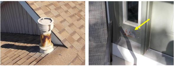
Rusted B-Vent and Paint on Front Door
