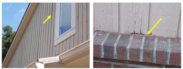
Examples of Weathered Siding with Opening Joints & Deterioration at Brick Ledge
