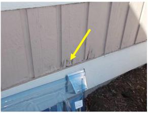
Deterioration at Water Table & Area of Rot
