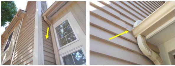
Rot at Gutter Ends (Kick-out flashing is recommended at roof and siding interfaces above these gutter ends)
