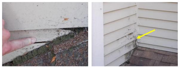
Rot at Roof Interface & Chimney Enclosure
