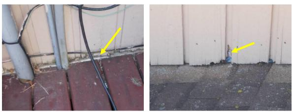
Deterioration at Deck & Roof Interfaces
