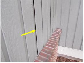
Examples of Deterioration and Open Joints
