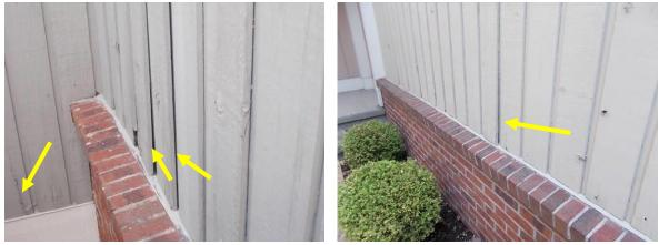
Opening Joints and Deterioration
