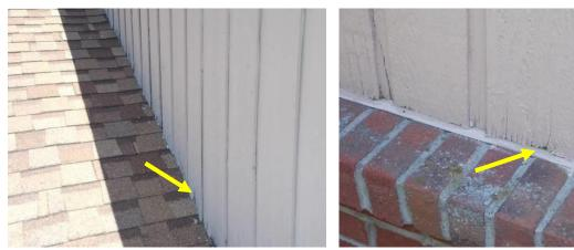
Examples of Deterioration at Brick and Roof Interfaces
