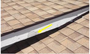
Roof Surface and Delaminating Paint on Trim
