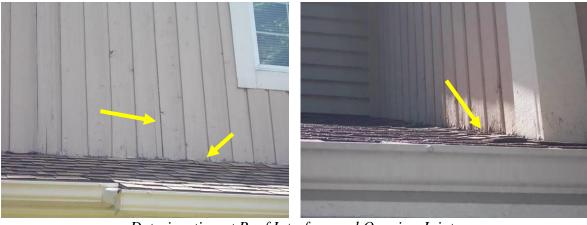
Deterioration at Roof Interface and Opening Joints
