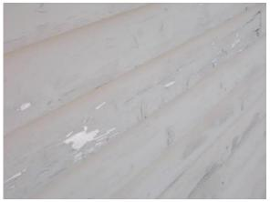
Missing Clapboard & Paint Delamination
