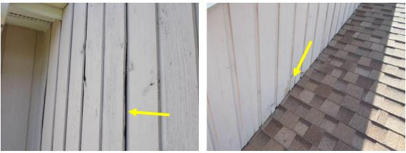
Opening Gap & Deterioration at Roof Surface
