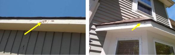
Examples of Deteriorated Trim & Insect (Carpenter Bee) Damage
