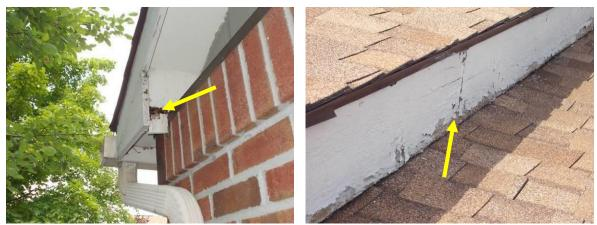
Examples of Damage and Deterioration to Trim in Need of Replacement
