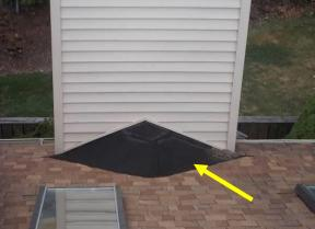
Example of Shingle Condition & Repaired Roof/Chimney Cricket
