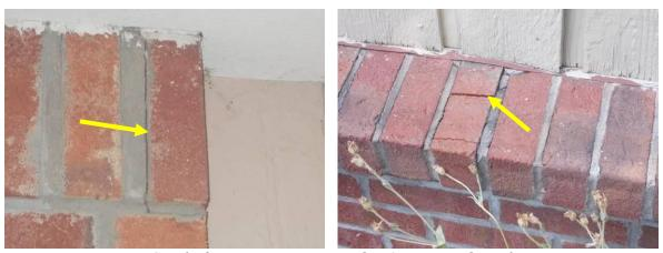
Cracked Mortar Joint at Header & Damaged Brick
