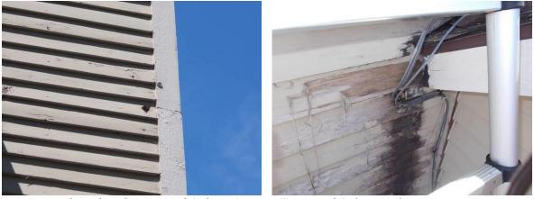
Weathered and Damaged Siding & Paint/Stain and Siding with Water Damage
