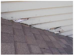
Deterioration to Siding on Chimney Enclosure and at Roof Interface
