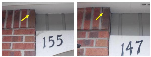
Examples of Cracked Mortar Joints at Garage Headers
