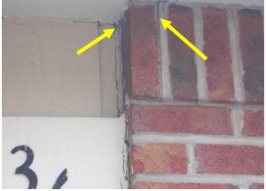
Cracking at Garage Header and Areas to Seal
