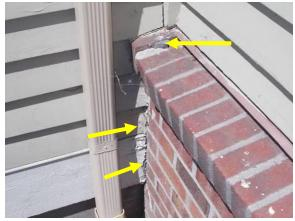
Damaged Brick with Deteriorated Siding and Trim
