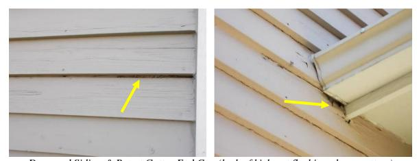
Damaged Siding & Rot at Gutter End Cap (lack of kick-out flashing above gutters)
