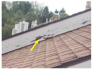
Examples of Trim Damage and Deterioration
