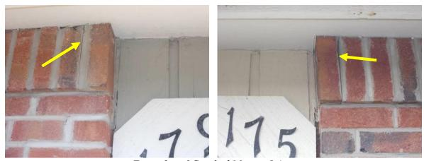
Examples of Cracked Mortar Joints
