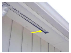
Gaps around Soffit Vent
