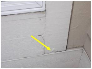
Examples of Damaged and Deteriorated Trim
