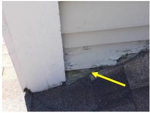
Examples of Deterioration to Clapboards
