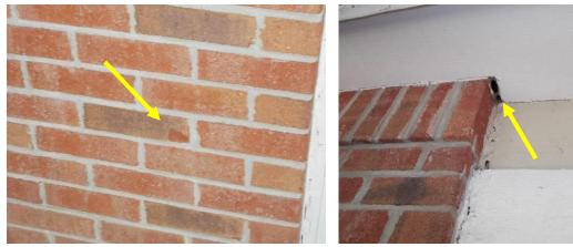
Spalled Brick & Area to Seal Around Brick Veneer
