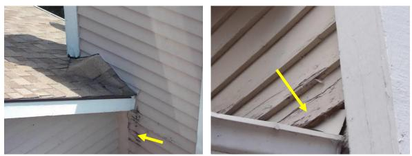
Examples of Deterioration to Siding and Paint/Stain
