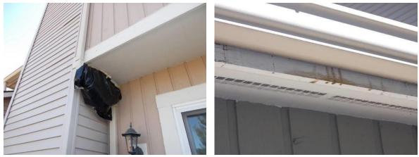
Gutter Downspout Wrapped in Garbage Bag & Staining Behind Gutter
