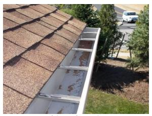
Roof Granules in Gutter
