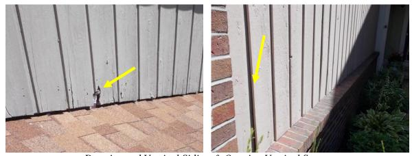
Deteriorated Vertical Siding & Opening Vertical Seams
