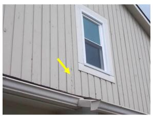
Opening Joints and Deterioration
