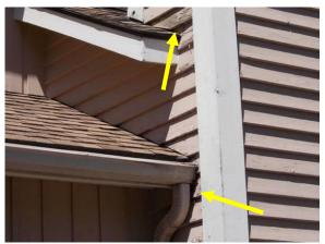
Examples of Deteriorated Clapboards
