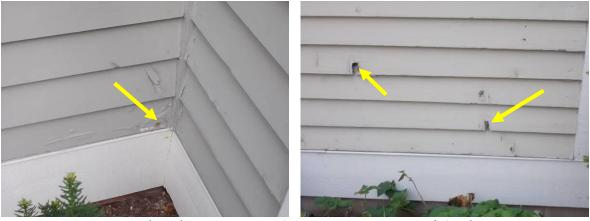
Examples of Deterioration & Damage Due to Wood Quality
