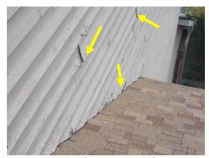
Wear and Damage to Siding
