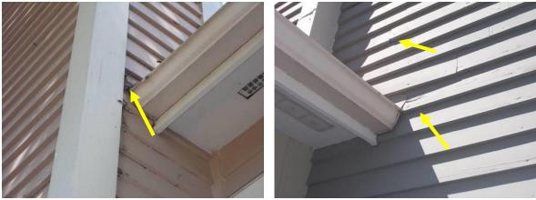
Deterioration and Cupping to Clapboards
