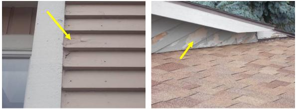
Clapboard Rot and Paint/Stain Delamination
