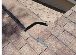
Roof Surface with Significant Granule Erosion
