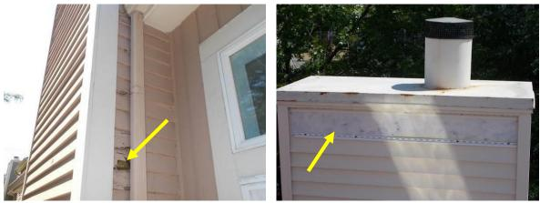
Water Damaged Clapboards & Missing Vinyl Siding on Chimney Enclosure
