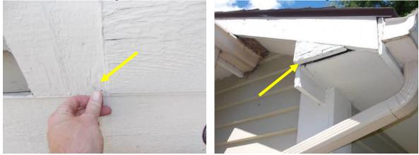
Examples of Rot Behind Coating & Damaged Trim with Gaps
