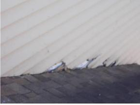
Examples of Deteriorated Clapboards
