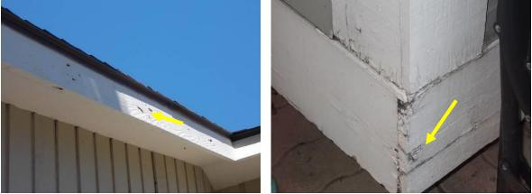
Insect Damage (Carpenter Bees) and Area of Deterioration at Chimney Enclosure
