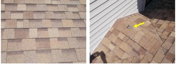
Example of Shingle Condition & Damaged Shingle on Chimney Cricket
