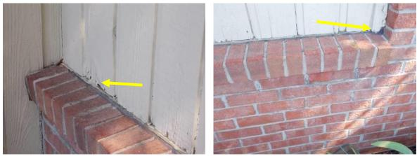
Rot and Deterioration at Water Table/Brick Ledge
