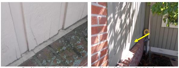
Cracking to Vertical Siding & Repair to Vertical Siding at Brick Ledge
