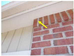
Cracked Mortar Joint
