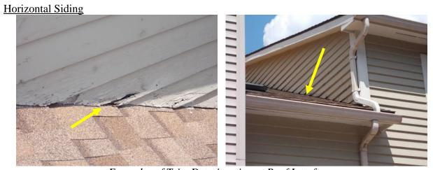
Examples of Trim Deterioration at Roof Interfaces
