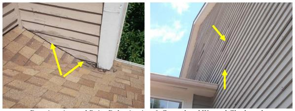
Deterioration and Paint Delamination & Cupped and Warped Clapboards
