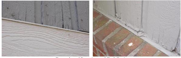
Examples of Deteriorated End Grain
