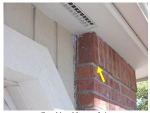
Cracking Mortar Joint
