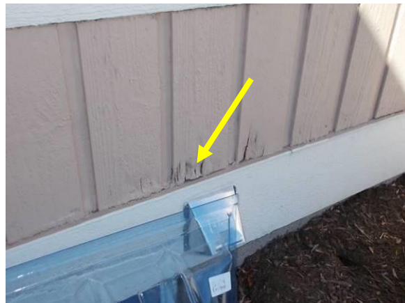
Deterioration at Water Table & Area of Rot
