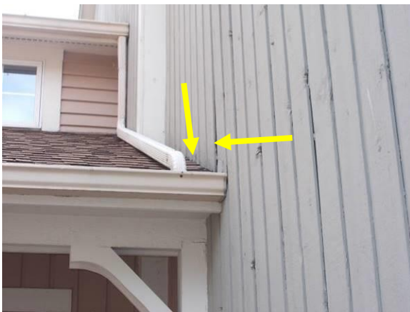
Examples of Deterioration and Open Joints
