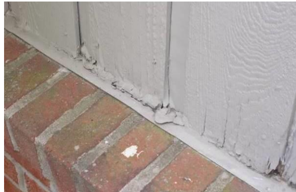
Examples of Deteriorated End Grain
