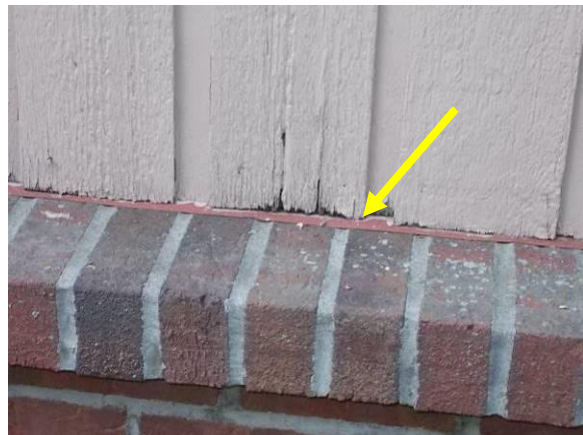
Examples of Weathered Siding with Opening Joints & Deterioration at Brick Ledge
