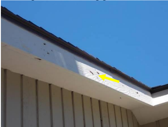
Insect Damage (Carpenter Bees) and Area of Deterioration at Chimney Enclosure
