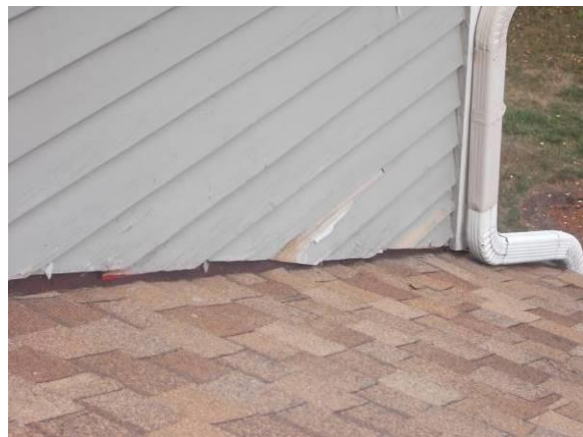
Examples of Delaminating Paint/Stain
