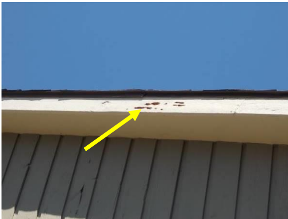
Examples of Deteriorated Trim & Insect (Carpenter Bee) Damage
