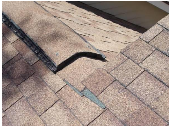
Roof Surface with Significant Granule Erosion
