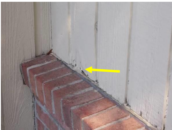
Rot and Deterioration at Water Table/Brick Ledge
