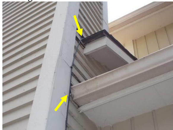
Water Damage To Chimney Enclosures
