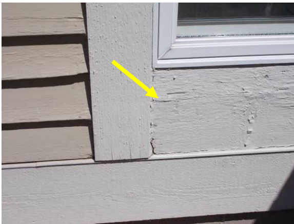
Examples of Deteriorated Trim
