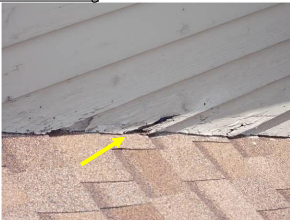
Examples of Trim Deterioration at Roof Interfaces
