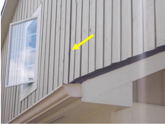
Gaps in Vertical Joints & Significant Damage at Roof Surfaces
