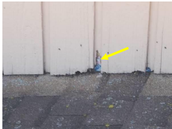
Deterioration at Deck & Roof Interfaces
