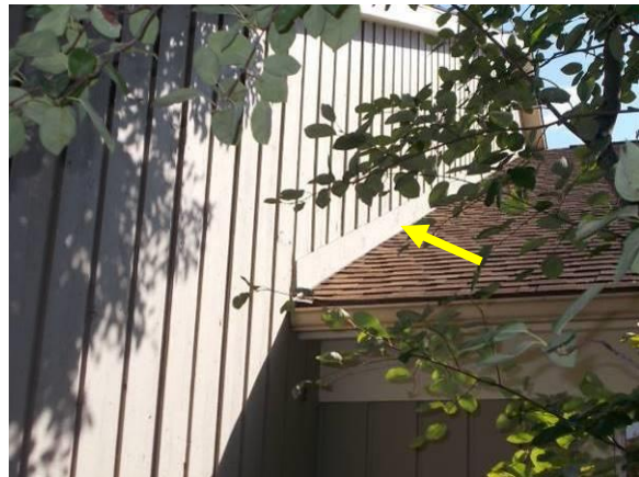
Deterioration at Brick Ledge & Repair to Lower Portion of Siding at Roof Surface
