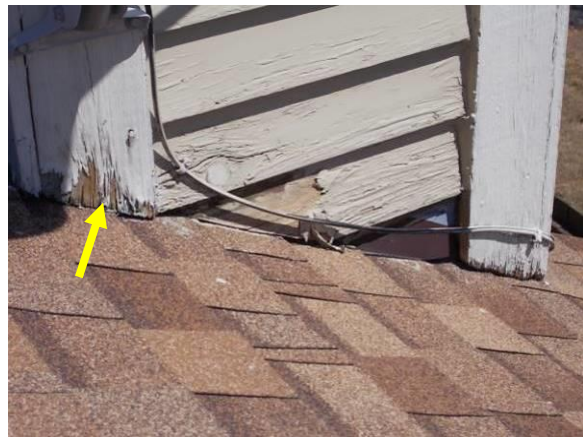
Examples of Deteriorated Trim
