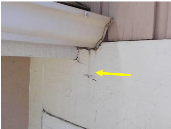
Trim Damaged from Leaking Gutter & Trim Damage at Chimney Enclosure
