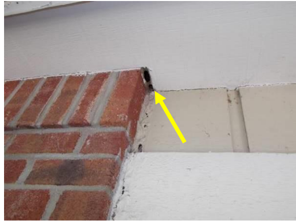
Spalled Brick & Area to Seal Around Brick Veneer
