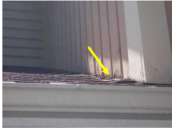
Deterioration at Roof Interface and Opening Joints
