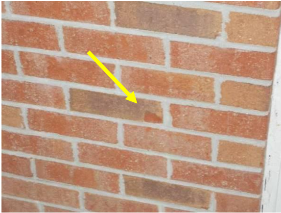
Spalled Brick & Area to Seal Around Brick Veneer
