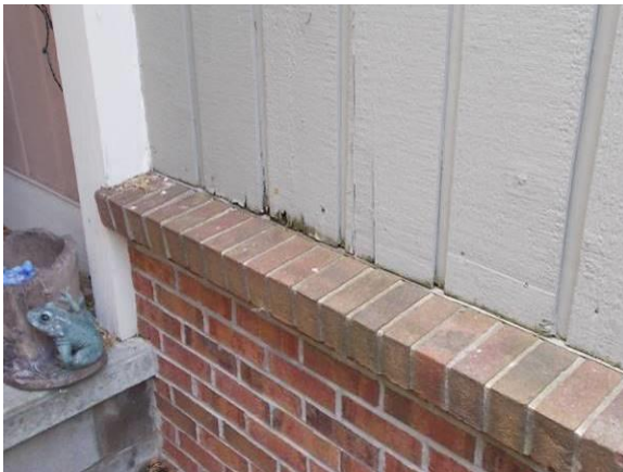
Deterioration at Brick Ledge & Repair to Lower Portion of Siding at Roof Surface
