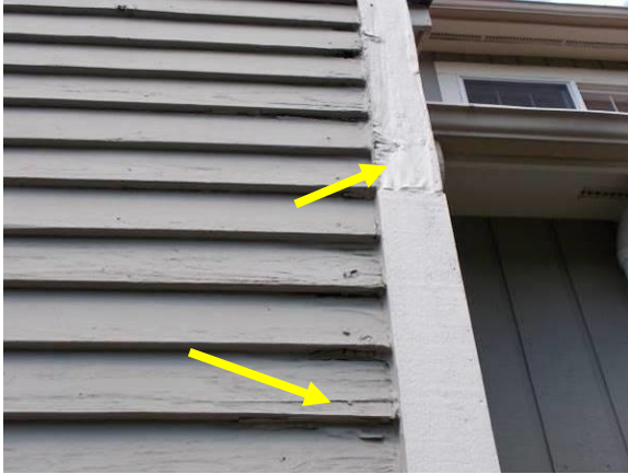
Rotted Trim and Severely Weathered Siding
