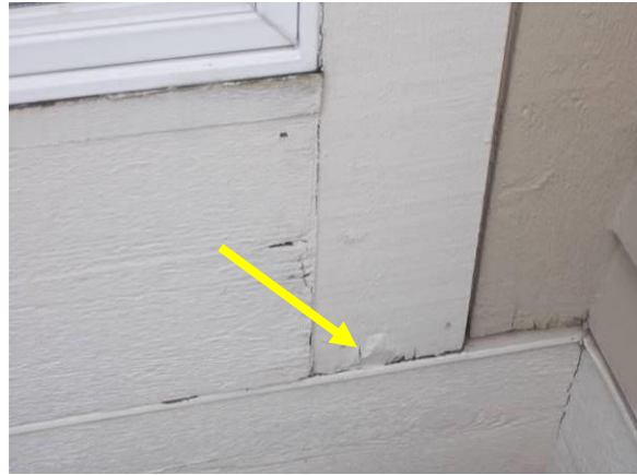
Examples of Damaged and Deteriorated Trim
