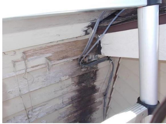
Weathered and Damaged Siding & Paint/Stain and Siding with Water Damage
