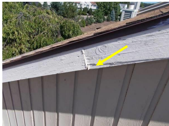
Examples of Trim Rot and Deterioration
