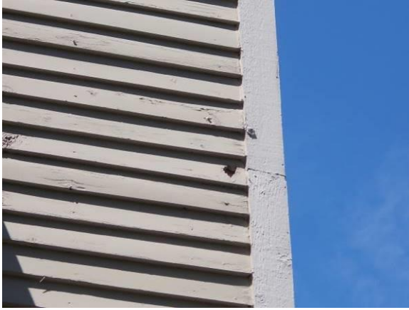
Weathered and Damaged Siding & Paint/Stain and Siding with Water Damage
