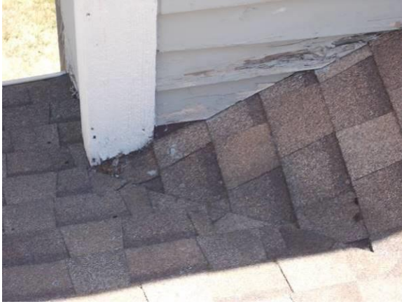
Examples of Deteriorated Clapboards
