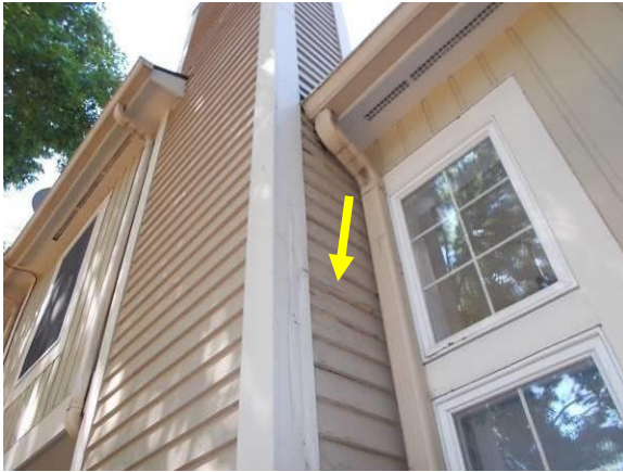
Rot at Gutter Ends
