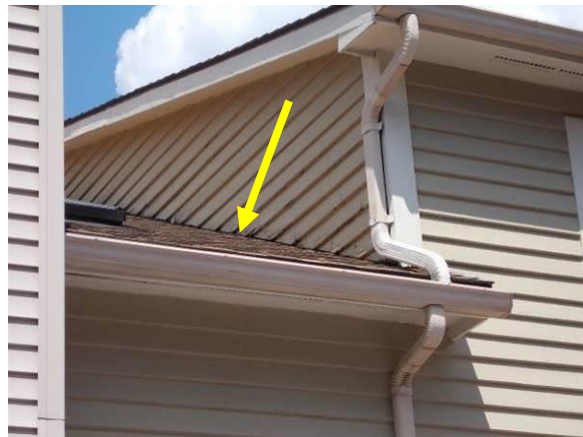
Examples of Trim Deterioration at Roof Interfaces
