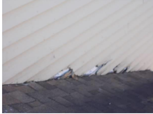
Examples of Deteriorated Clapboards
