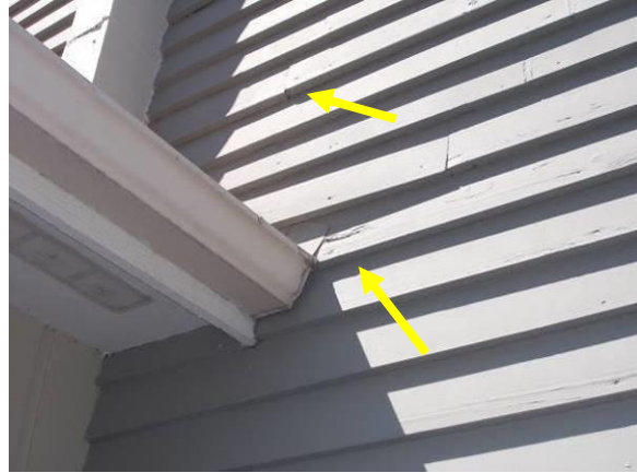
Deterioration and Cupping to Clapboards
