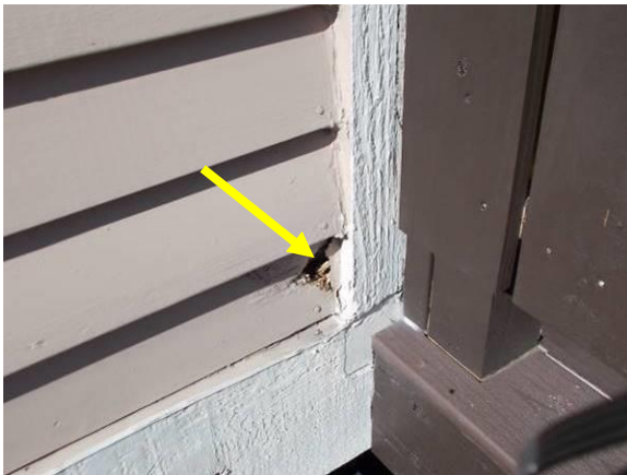
Rot in Clapboards
