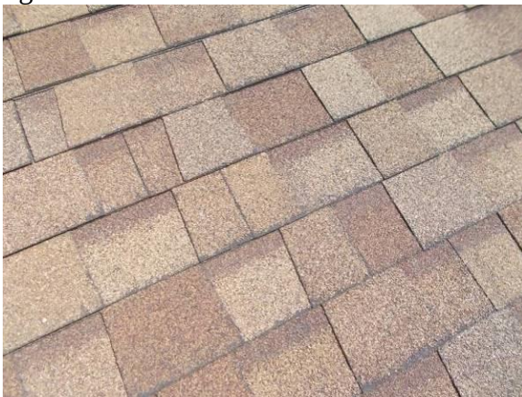
Example of Worn Shingle Surfaces and a Missing Shingle Tab/Edge
