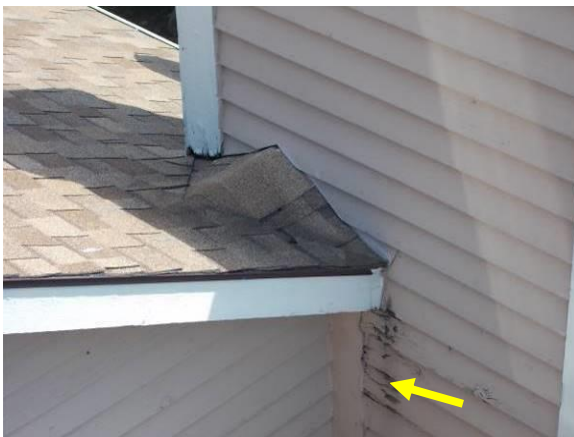
Examples of Deterioration to Siding and Paint/Stain
