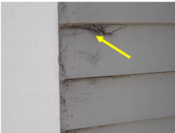
Examples of Deteriorated Clapboards
