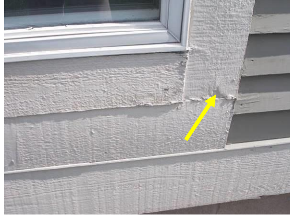
Examples of Trim Deterioration
