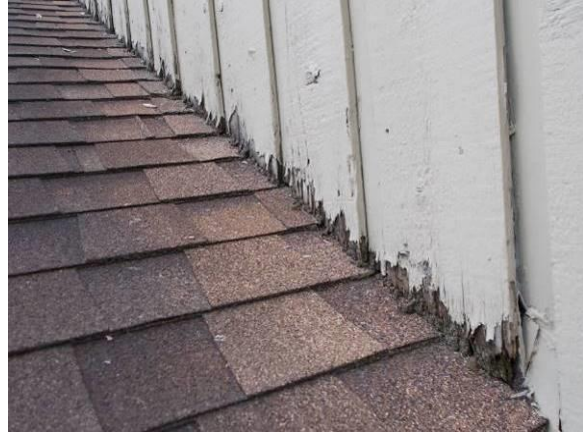
Gaps in Vertical Joints & Significant Damage at Roof Surfaces
