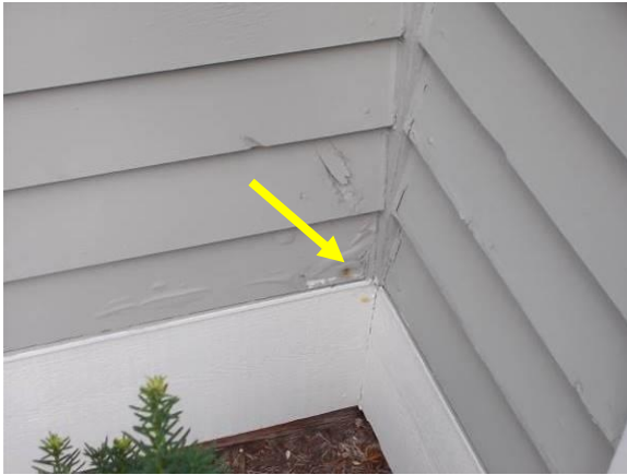
Examples of Deterioration & Damage Due to Wood Quality
