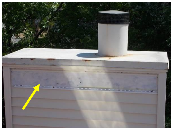
Water Damaged Clapboards & Missing Vinyl Siding on Chimney Enclosure
