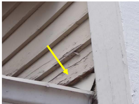
Examples of Deterioration to Siding and Paint/Stain
