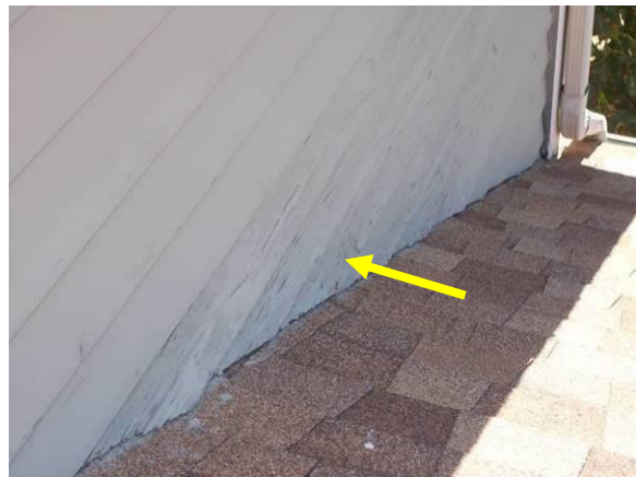
Examples of Deterioration to Clapboards
