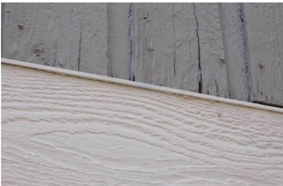
Examples of Deteriorated End Grain
