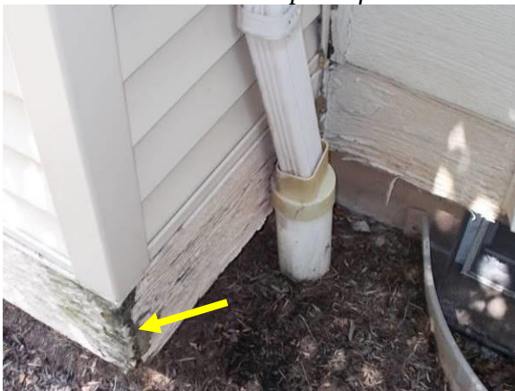
Examples of Rot in Trim & Insect Damage (Carpenter Bees)
