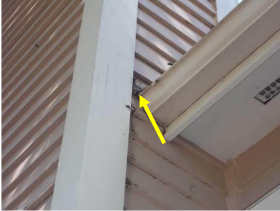
Deterioration and Cupping to Clapboards
