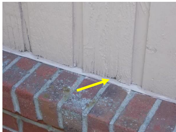
Examples of Deterioration at Brick and Roof Interfaces
