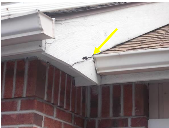
Examples of Trim Damage and Deterioration
