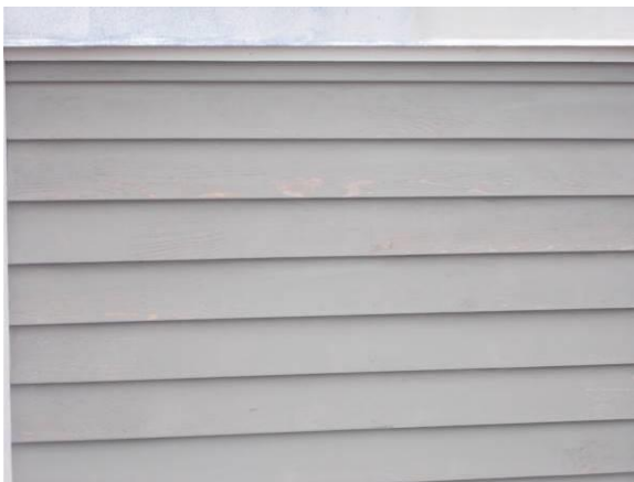
Examples of Delaminating Paint/Stain
