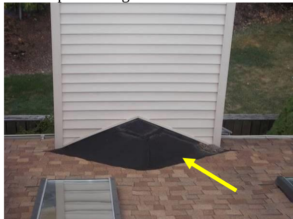
Example of Shingle Condition & Repaired Roof/Chimney Cricket
