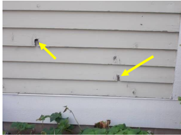
Examples of Deterioration & Damage Due to Wood Quality
