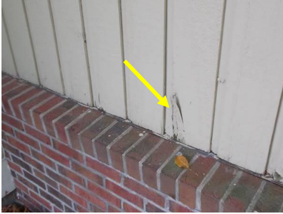
Examples of Deterioration and Open Joints
