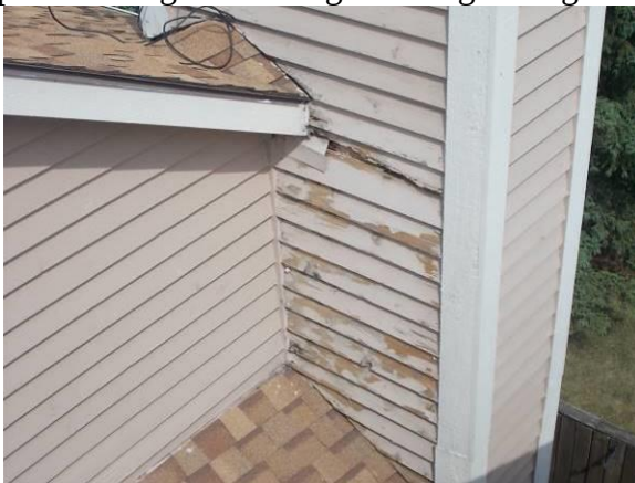
Water Damage To Chimney Enclosures
