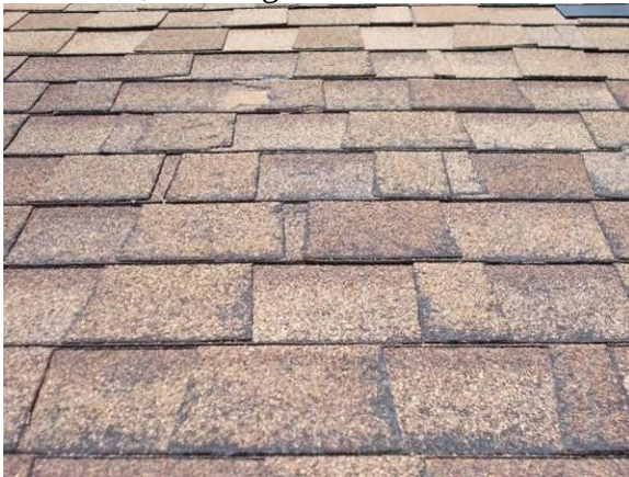
Roof Surface with Significant Granule Erosion
