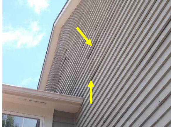
Deterioration and Paint Delamination & Cupped and Warped Clapboards
