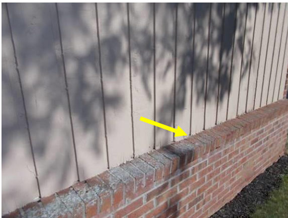
Deterioration at Water Table & Area of Rot
