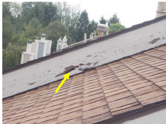
Examples of Trim Damage and Deterioration
