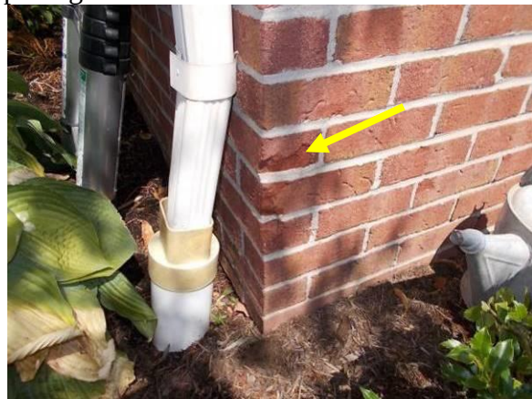
Damaged Bricks
