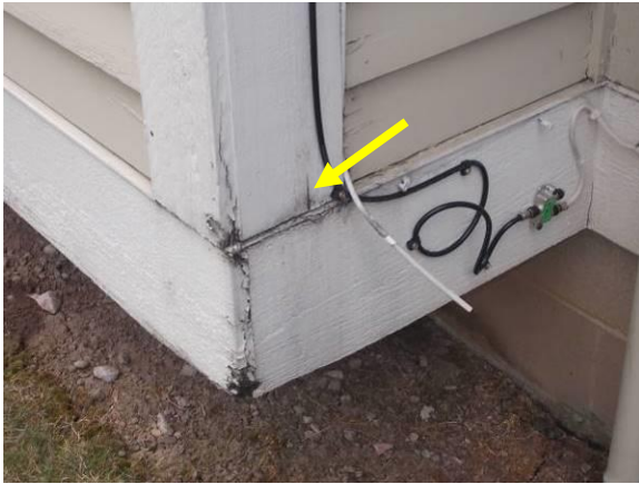
Examples of Trim Damage and Deterioration
