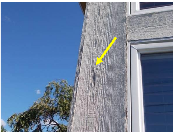
Examples of Trim Rot and Deterioration
