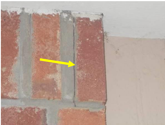
Cracked Mortar Joint at Header & Damaged Brick
