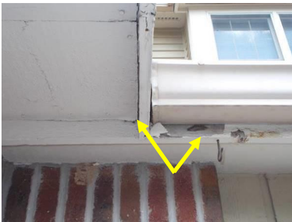
Examples of Trim Deterioration
