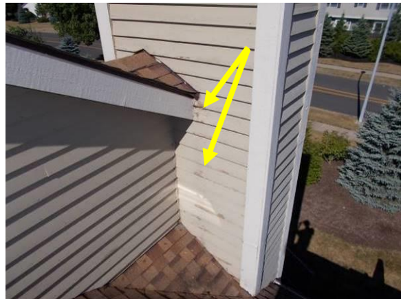
Rot in Clapboards
