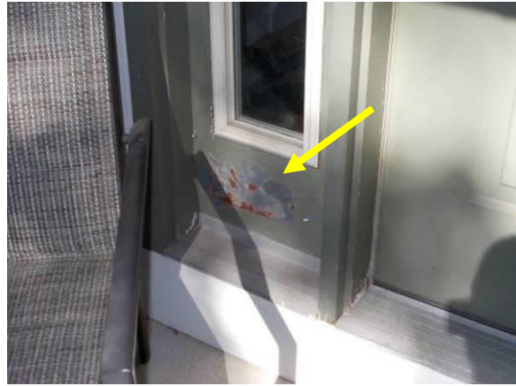
Rusted B-Vent and Paint on Front Door
