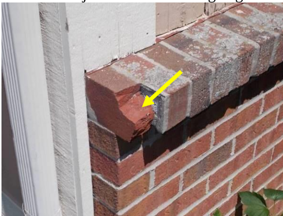
Damaged Bricks
