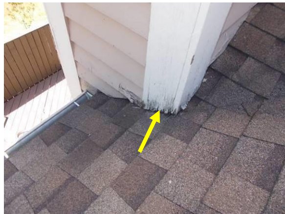
Examples of Deteriorated Trim
