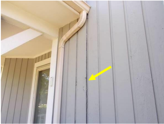
Open Seam in Vertical Siding & Deteriorated Siding and Trim
