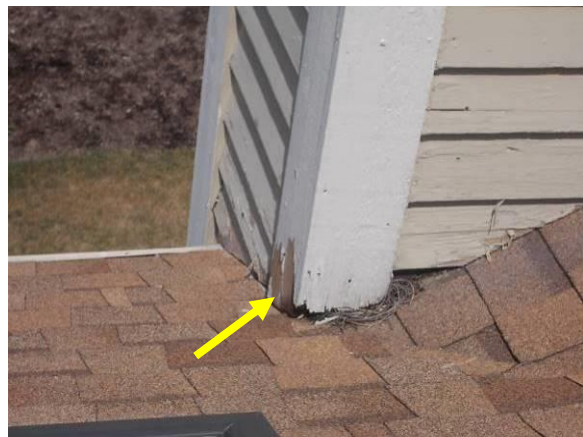
Examples of Trim Deterioration
