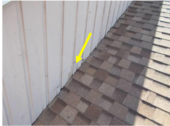
Opening Gap & Deterioration at Roof Surface
