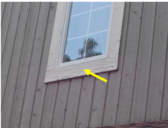
Examples of Rot in Need of Repair and Gaps in Trim
