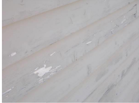
Missing Clapboard & Paint Delamination
