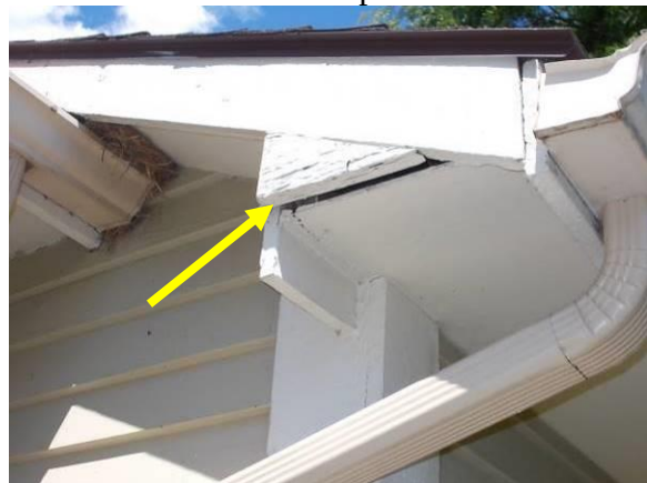
Examples of Rot Behind Coating & Damaged Trim with Gaps
