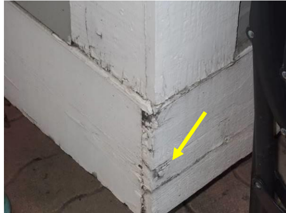
Insect Damage (Carpenter Bees) and Area of Deterioration at Chimney Enclosure
