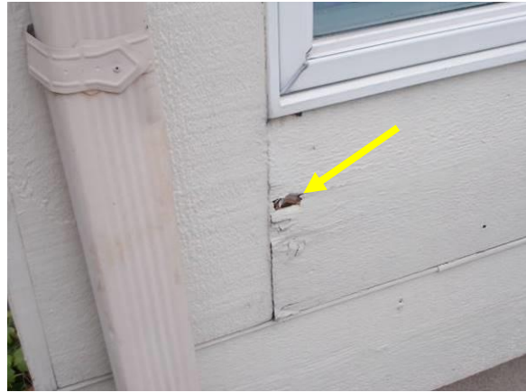
Examples of Damage to Trim and Paint/Stain
