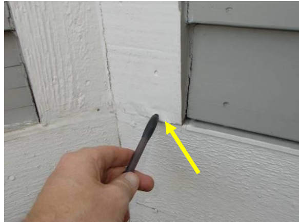
Cracking Mortar Joint
