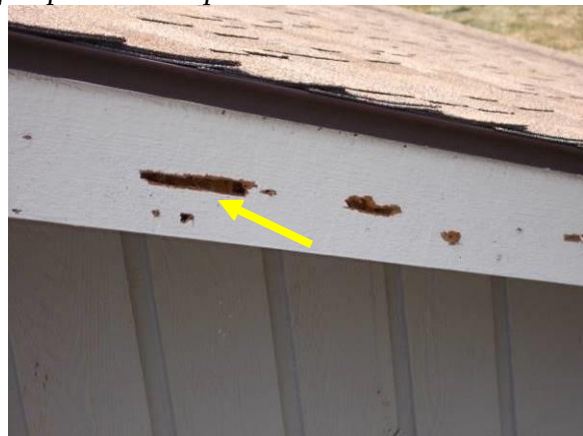
Examples of Rot in Trim & Insect Damage (Carpenter Bees)
