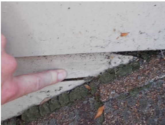
Rot at Roof Interface & Chimney Enclosure
