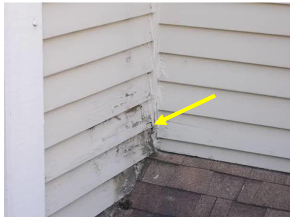
Rot at Roof Interface & Chimney Enclosure
