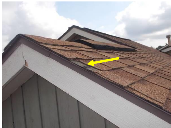
Example of Worn Shingle Surfaces and a Missing Shingle Tab/Edge
