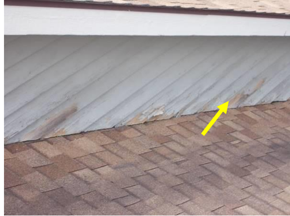
Rotted Trim and Severely Weathered Siding
