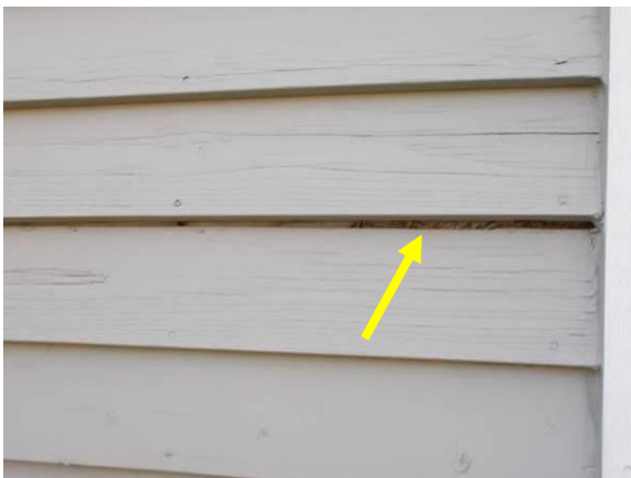
Damaged Siding & Rot at Gutter End Cap (lack of kick-out flashing above gutters)
