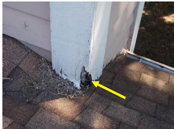
Trim Damaged from Leaking Gutter & Trim Damage at Chimney Enclosure
