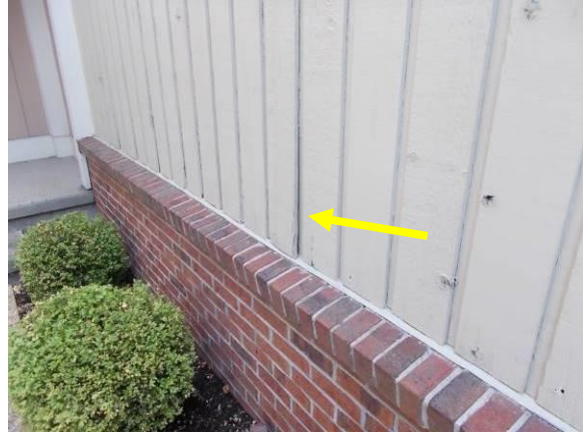
Opening Joints and Deterioration
