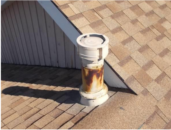
Rusted B-Vent and Paint on Front Door
