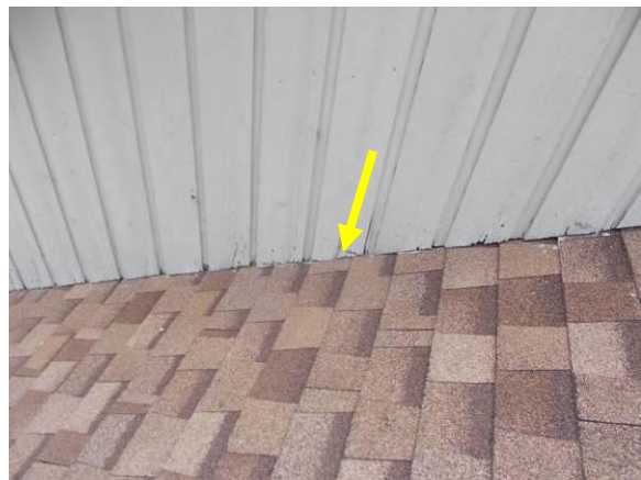
Examples of Deterioration and Open Joints
