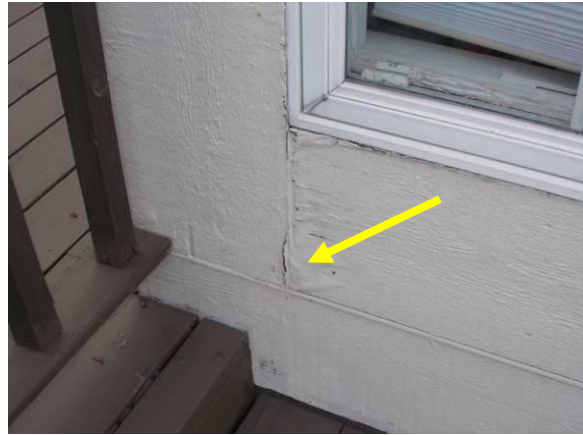
Examples of Trim Damage and Deterioration
