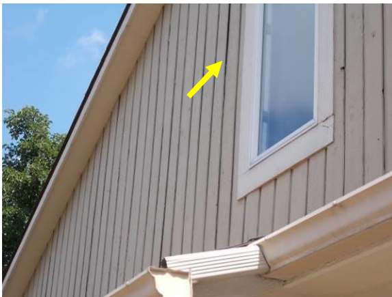
Examples of Weathered Siding with Opening Joints & Deterioration at Brick Ledge
