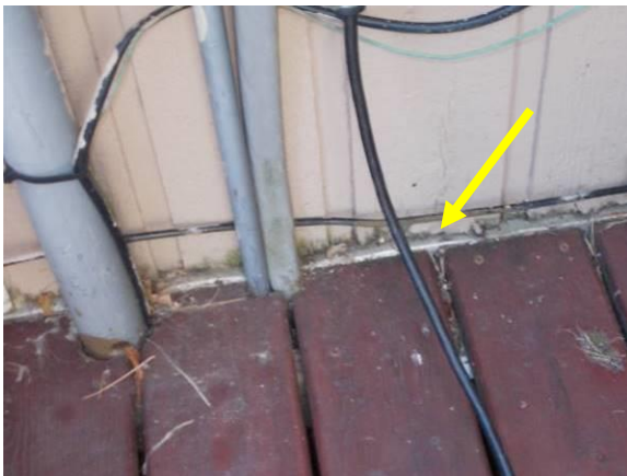
Deterioration at Deck & Roof Interfaces
