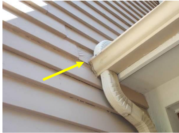
Rot at Gutter Ends
