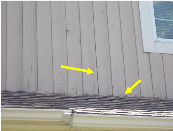
Deterioration at Roof Interface and Opening Joints
