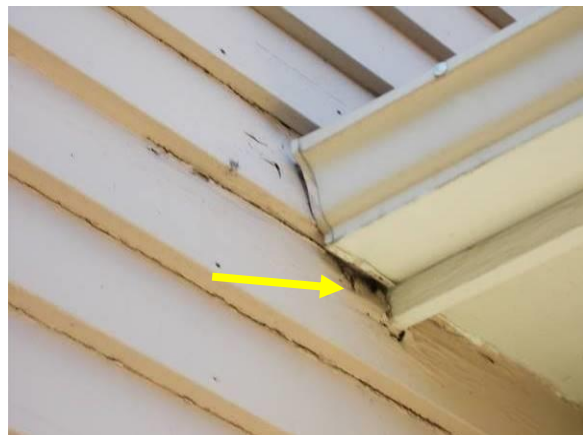
Damaged Siding & Rot at Gutter End Cap (lack of kick-out flashing above gutters)
