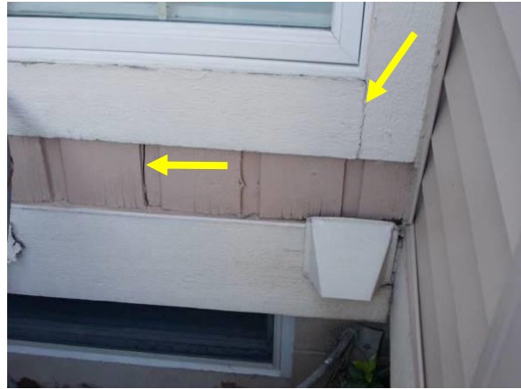
Open Seam in Vertical Siding & Deteriorated Siding and Trim
