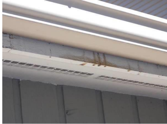
Gutter Downspout Wrapped in Garbage Bag & Staining Behind Gutter
