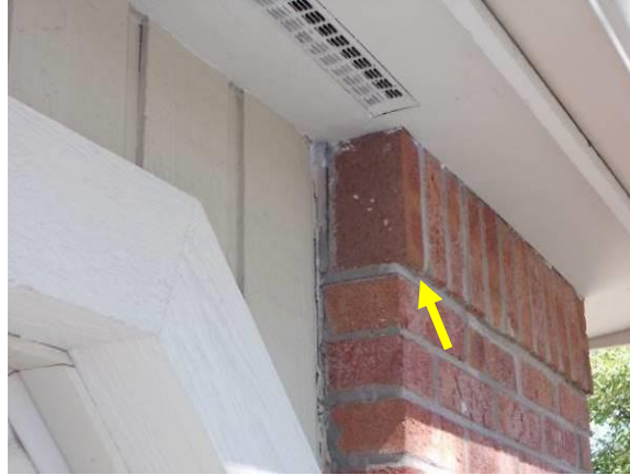
Cracking Mortar Joint
