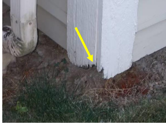
Trim with Rot and Damage
