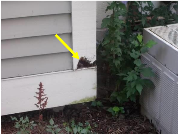
Examples of Damaged and Deteriorated Trim
