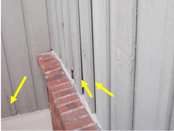
Opening Joints and Deterioration
