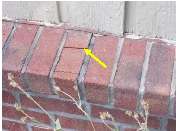
Cracked Mortar Joint at Header & Damaged Brick
