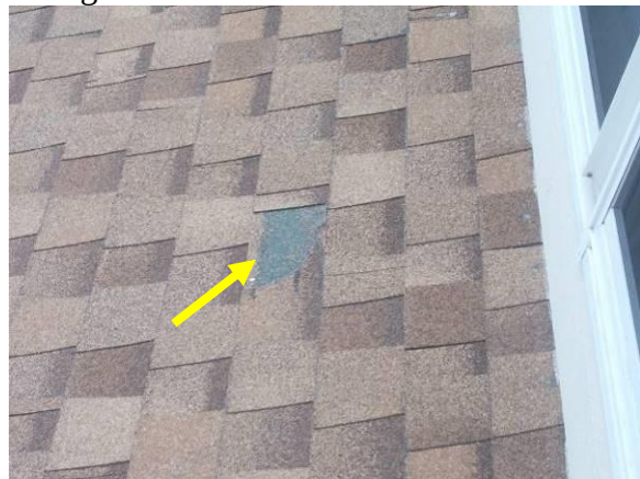
Roof Surface and Damaged Shingle
