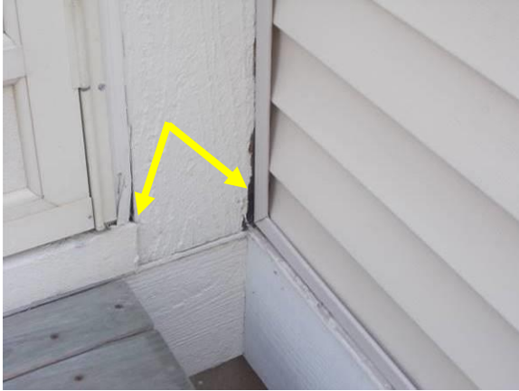
Examples of Trim Deterioration
