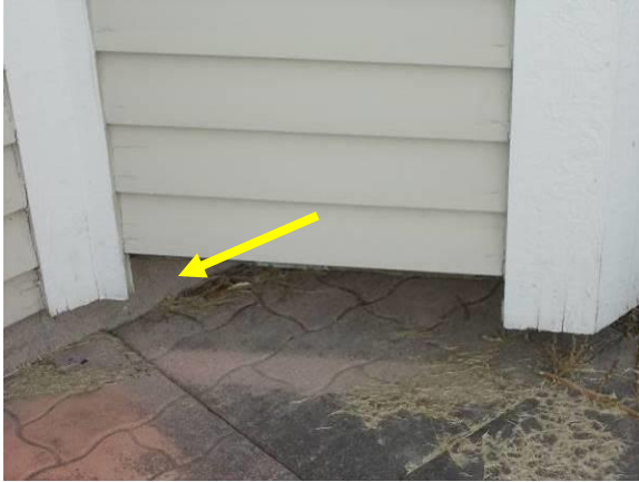
Missing Clapboard & Paint Delamination
