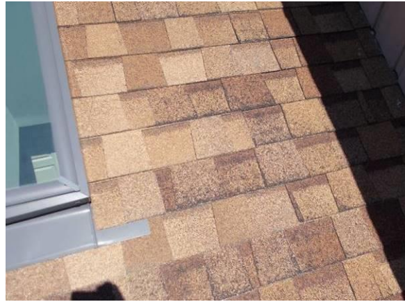
Example of Roof Condition (Advanced Wear on this Building)
