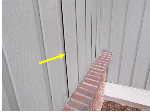
Examples of Deterioration and Open Joints
