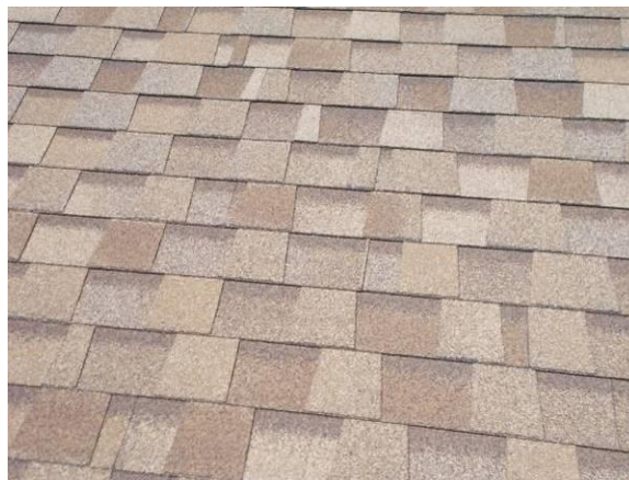
Example of Roof Surface
