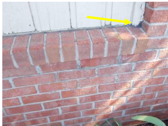
Rot and Deterioration at Water Table/Brick Ledge
