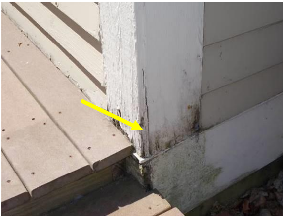
Examples of Deteriorated Trim
