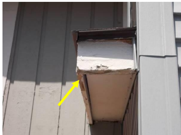
Examples of Rot in Need of Repair and Gaps in Trim
