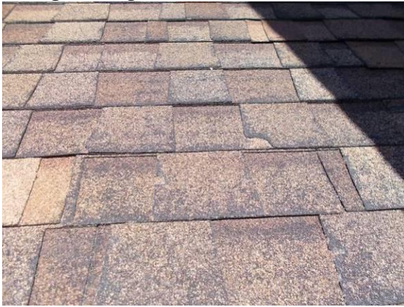
Example of Roof Condition (Advanced Wear on this Building)
