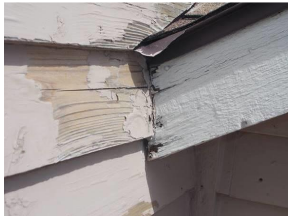
Examples of Water Damage
