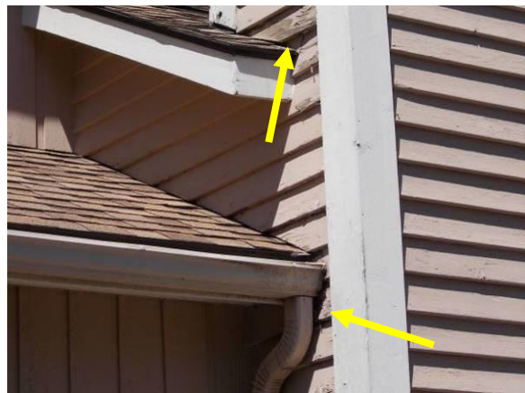
Examples of Deteriorated Clapboards
