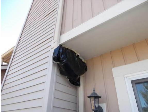
Gutter Downspout Wrapped in Garbage Bag & Staining Behind Gutter
