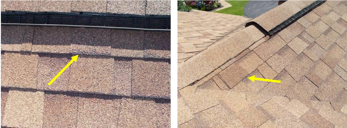
Examples of Roof Wear
