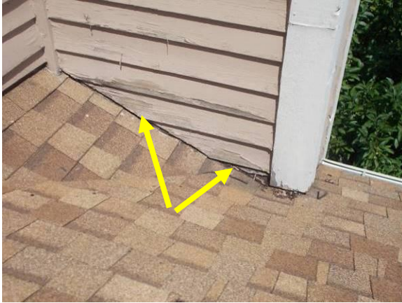
Deterioration and Paint Delamination & Cupped and Warped Clapboards
